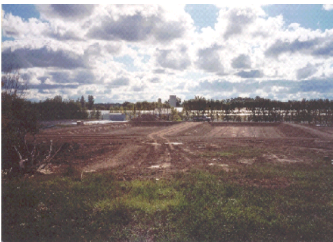
excavation for 6 cells.....
